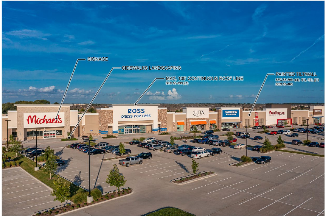
The image shows the elevations for the “big box” retail, compliant with the I-35 Overlay.
