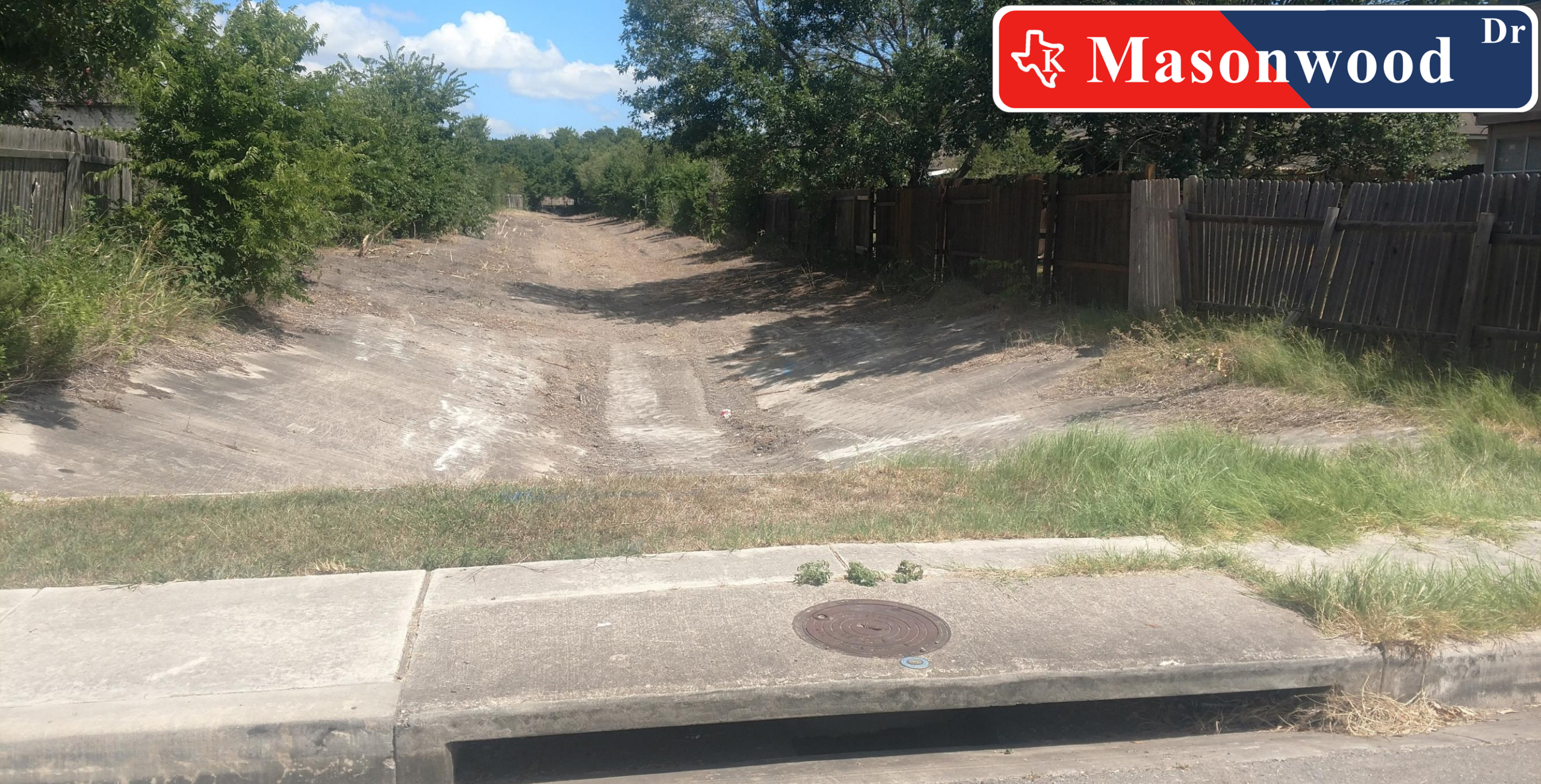
Upstream inlet at Masonwood Dr. – channel restoration
