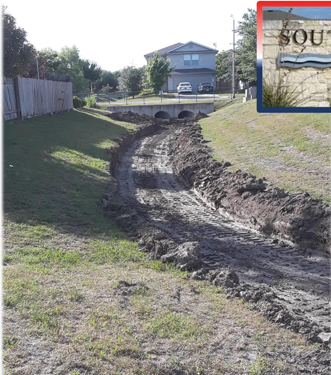
Restoring channel depth and grade
