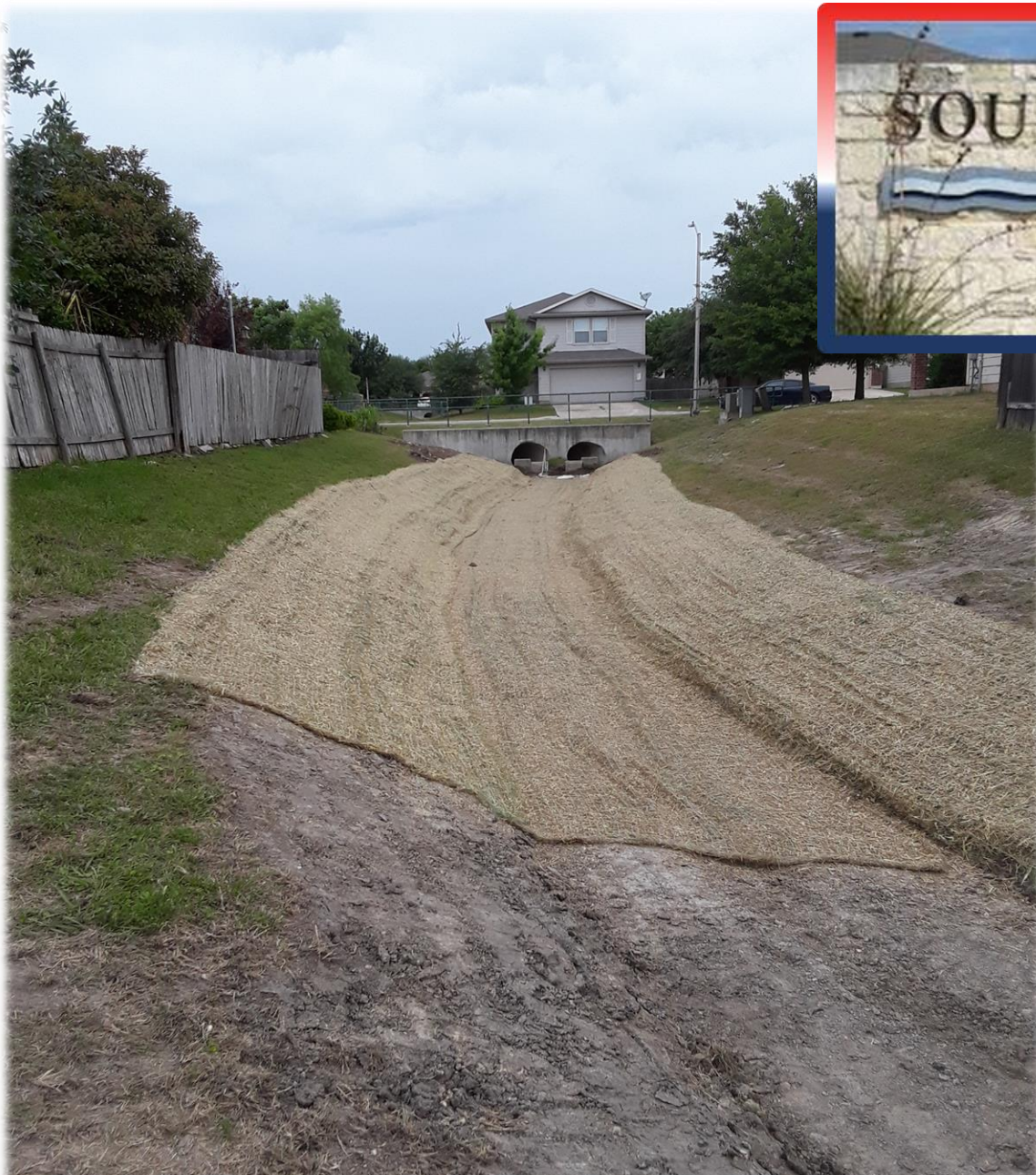
Installing revegetative matting
