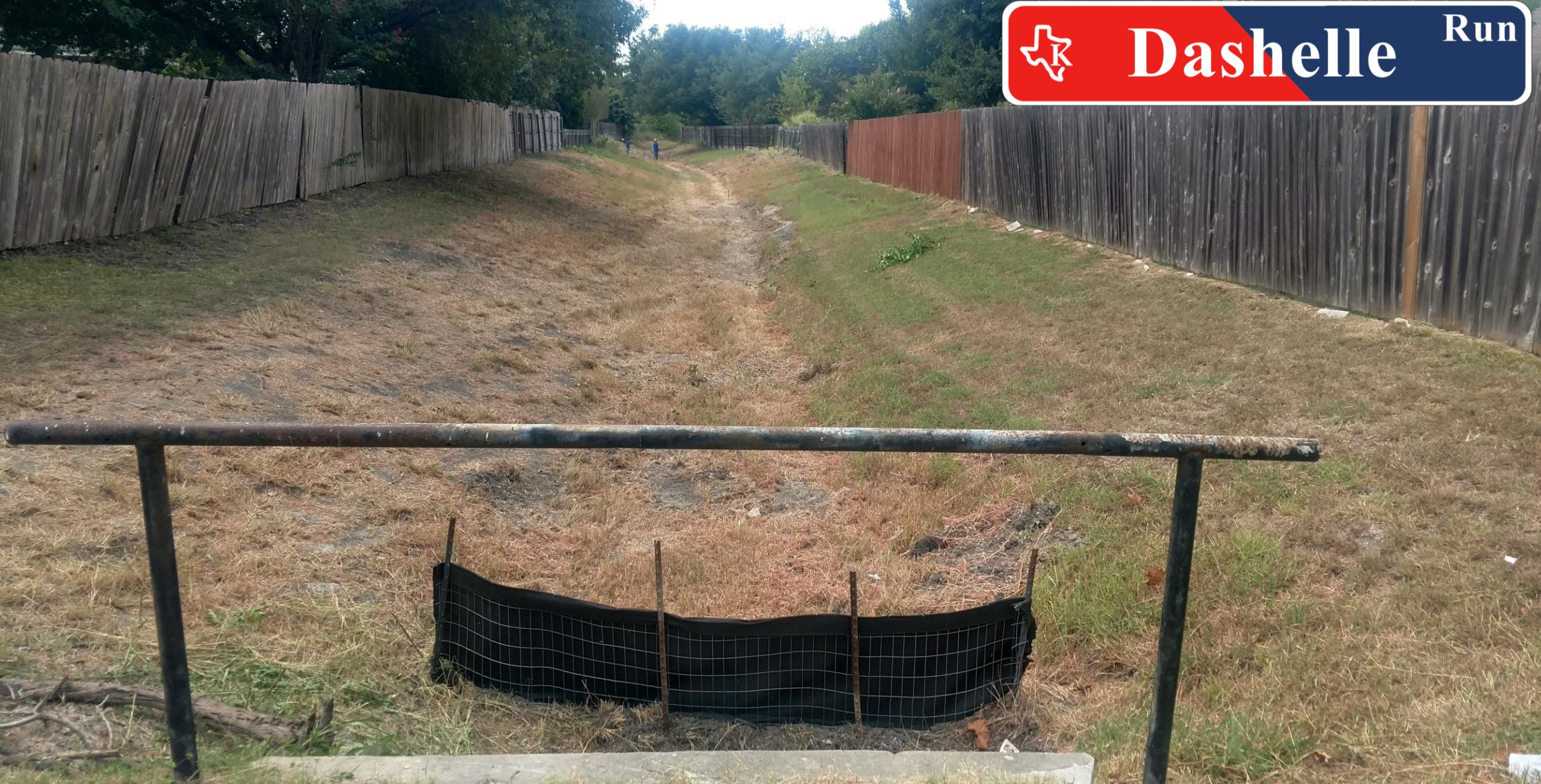
Dashelle Run – upstream SE inlet after maintenance
