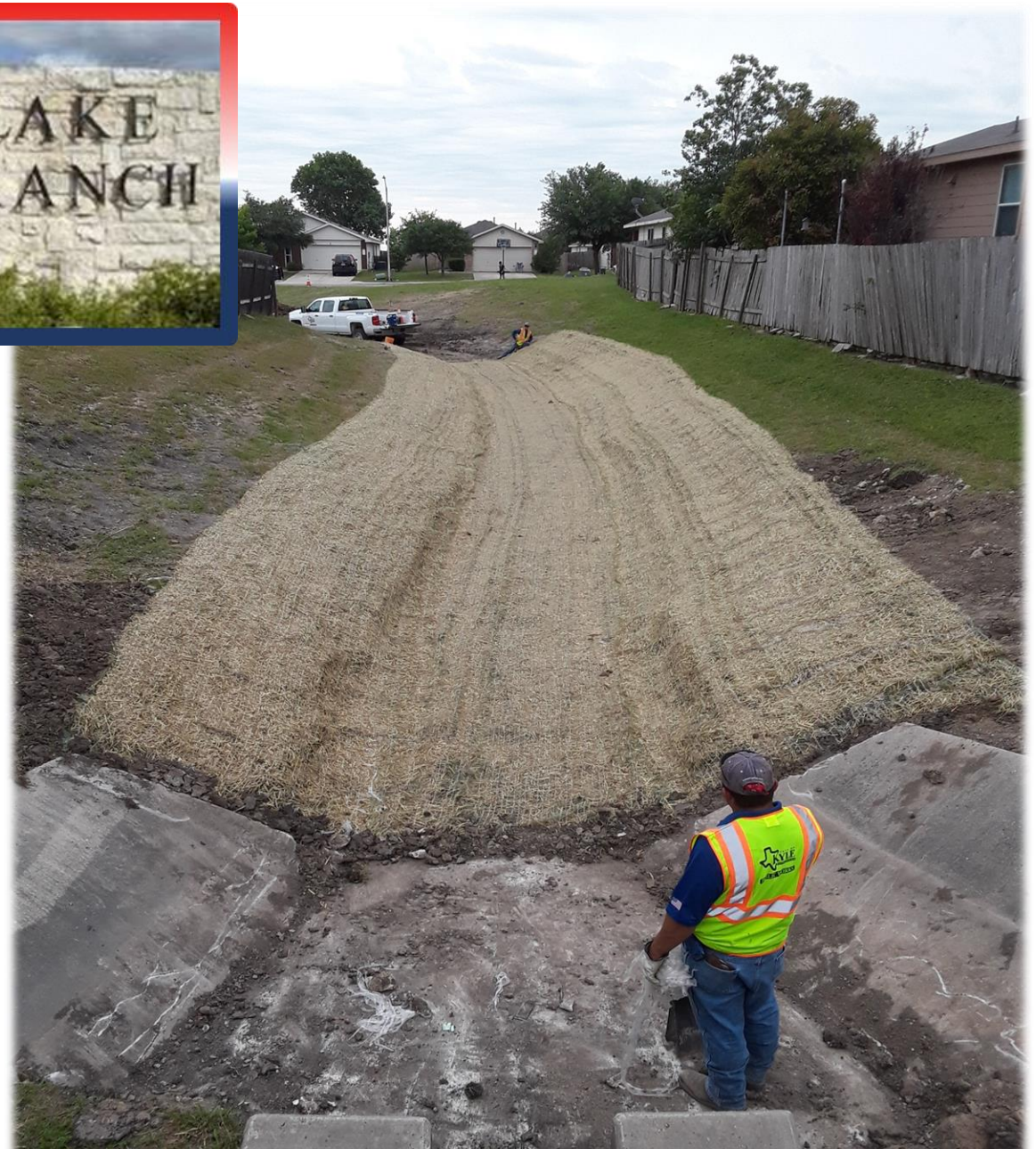
Installing revegetative matting
