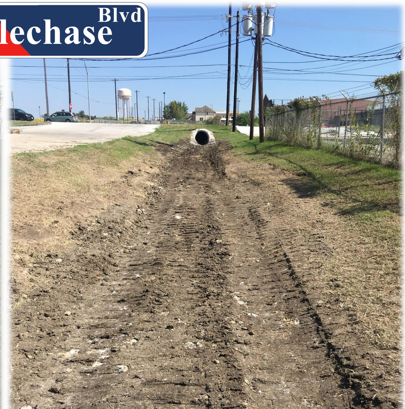
Facing upstream towards Bunton Creek Rd. – channel regrading 25
