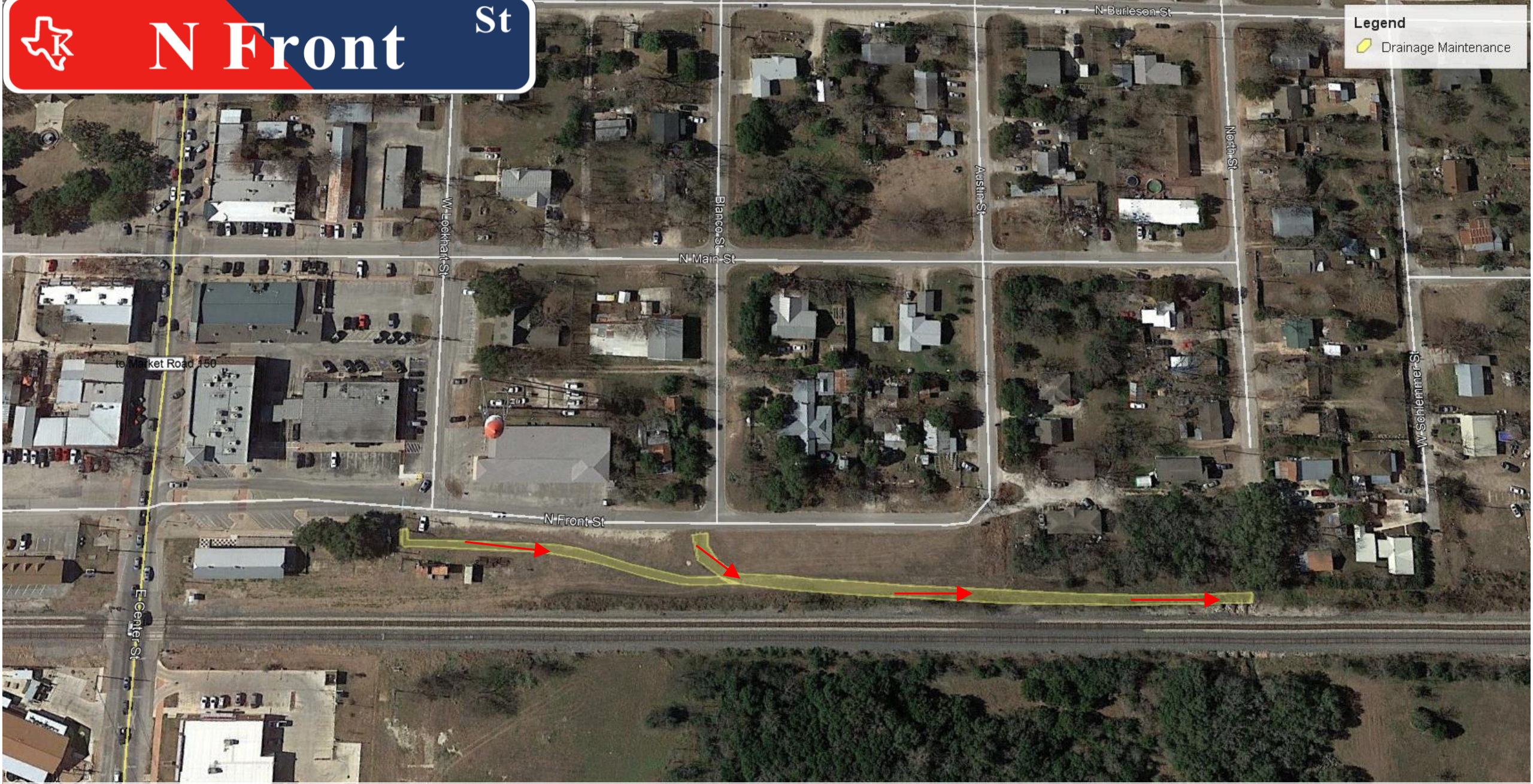
Front Street channel regrading from Lockhart St to North St
