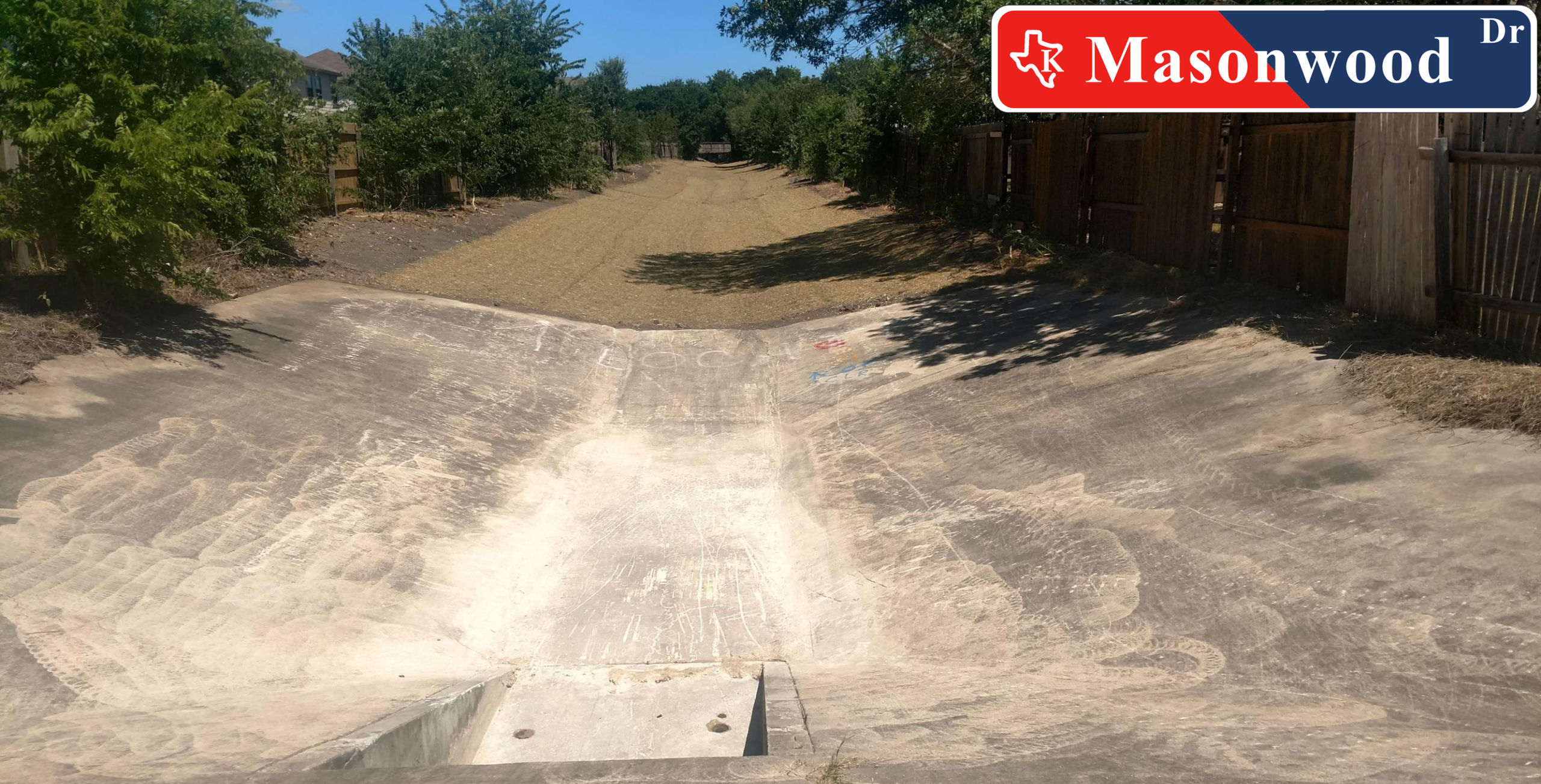
Upstream inlet at Masonwood Dr. – final revegetation
