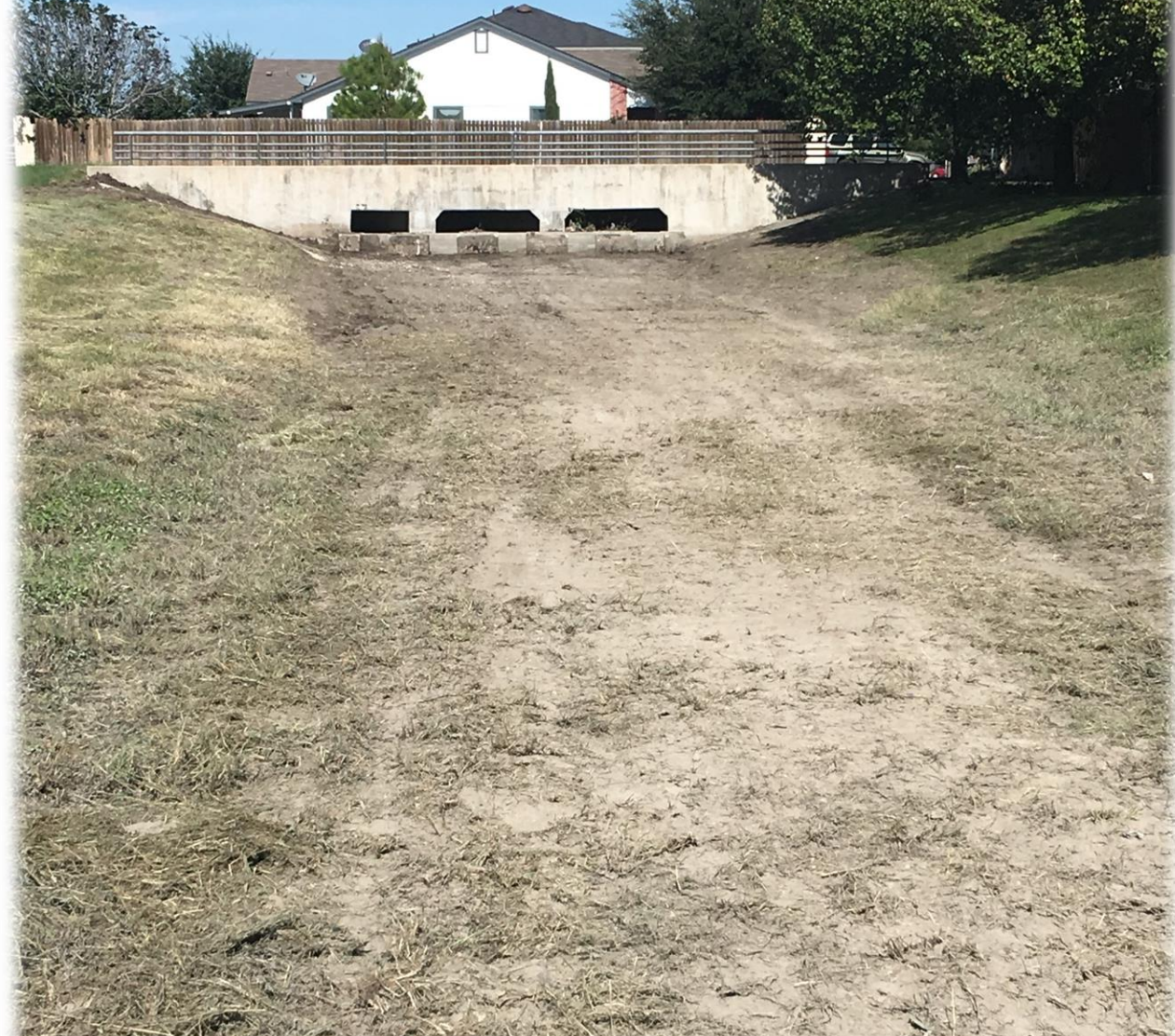
Facing upstream towards Brent Blvd. – channel regrading
