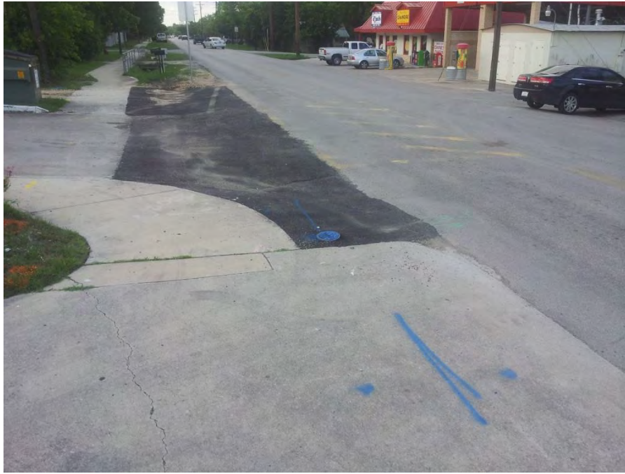
Photo 1 – Boring B-1 near W. Center Street, facing north.
