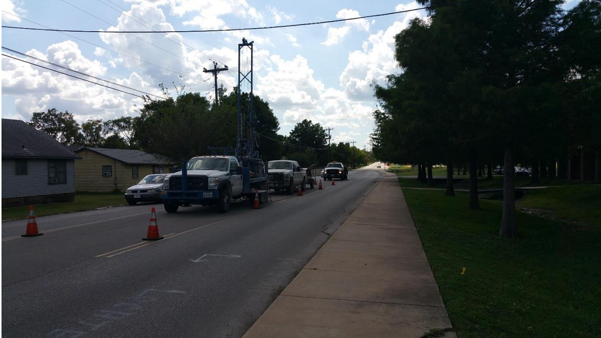
Photo 1 (8/5/16) – Drilling B-3, facing west
