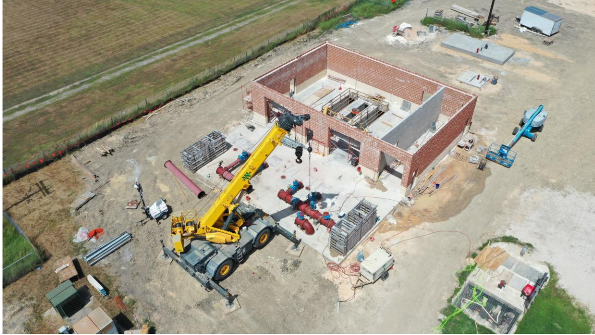
Headworks Walls Completed
