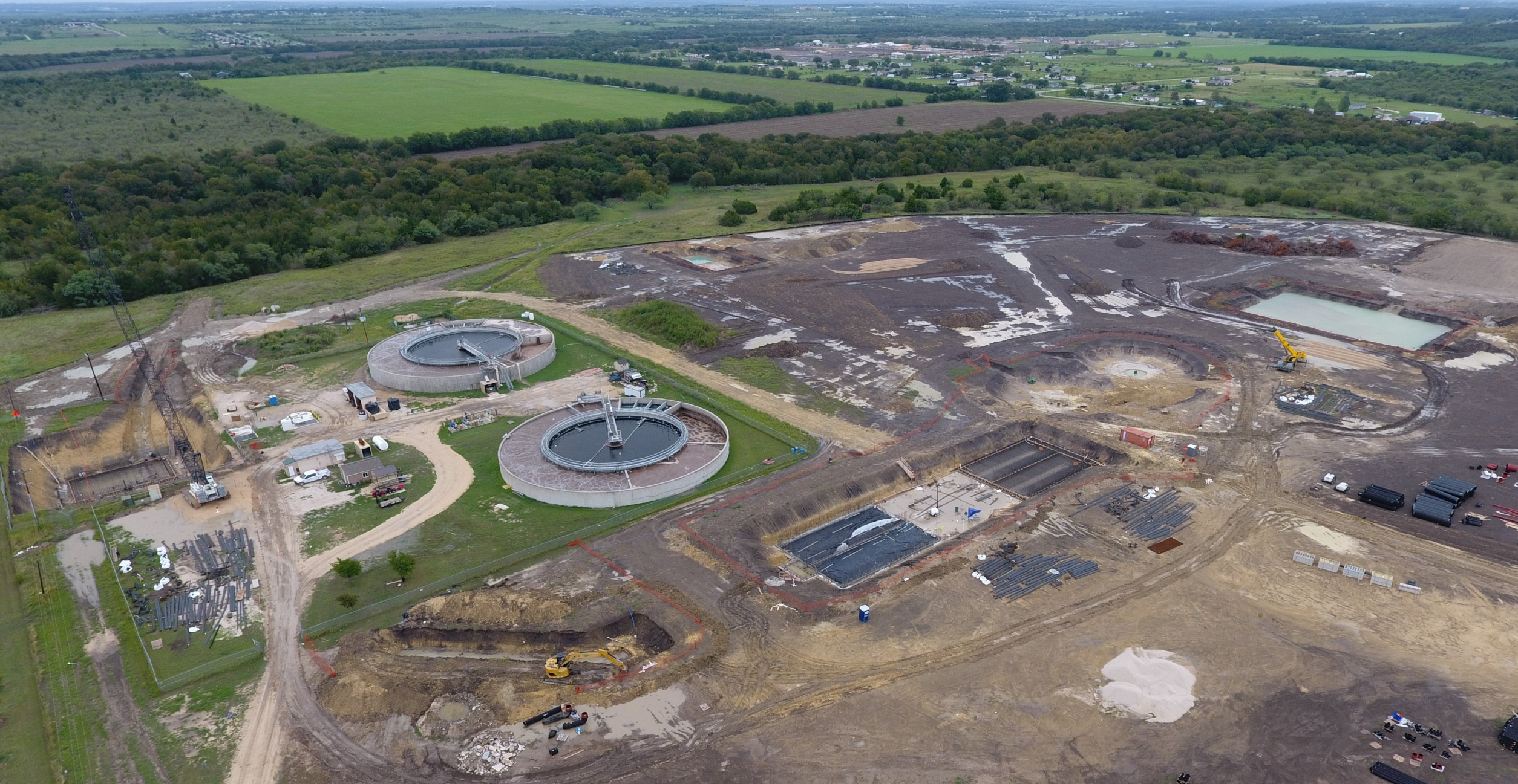
WWTP Expansion - September 10, 2020 Rain Accumulation
