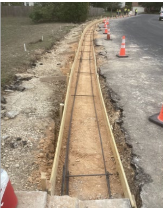
Preparation for Sidewalk, Curb, and Gutter Installation
