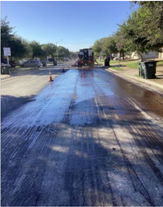
Preparing Milled Surface for Overlay
