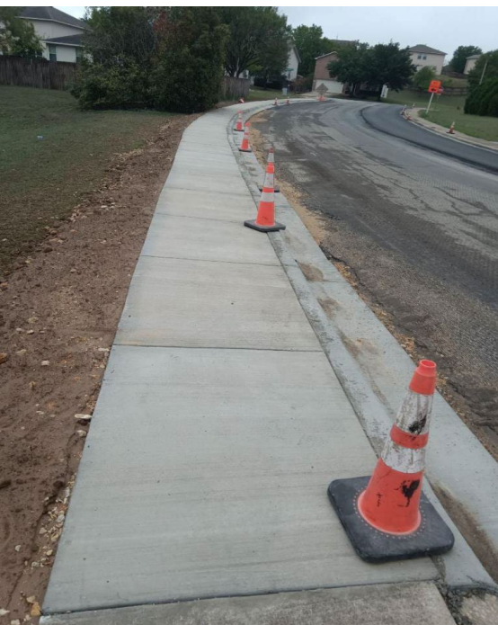
Curb, Gutter, and Sidewalk Complete (East Side)
