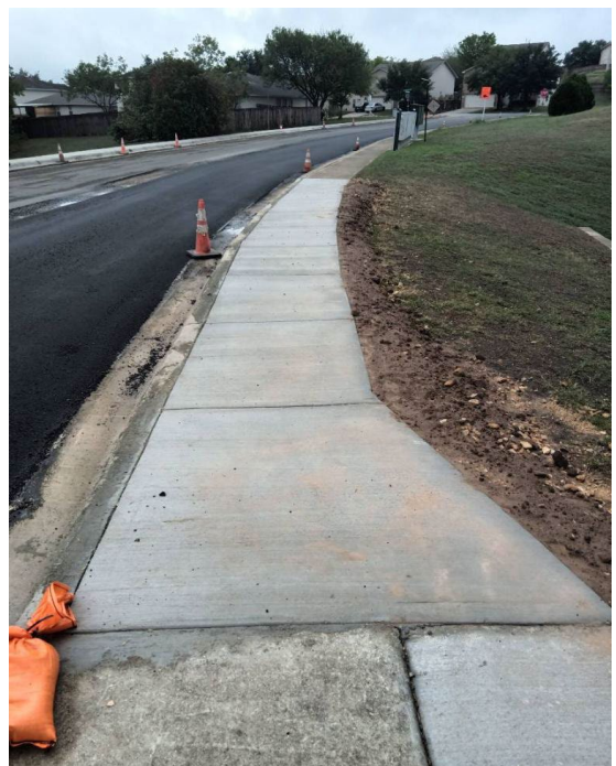
Curb, Gutter, and Sidewalk Complete (West Side)
