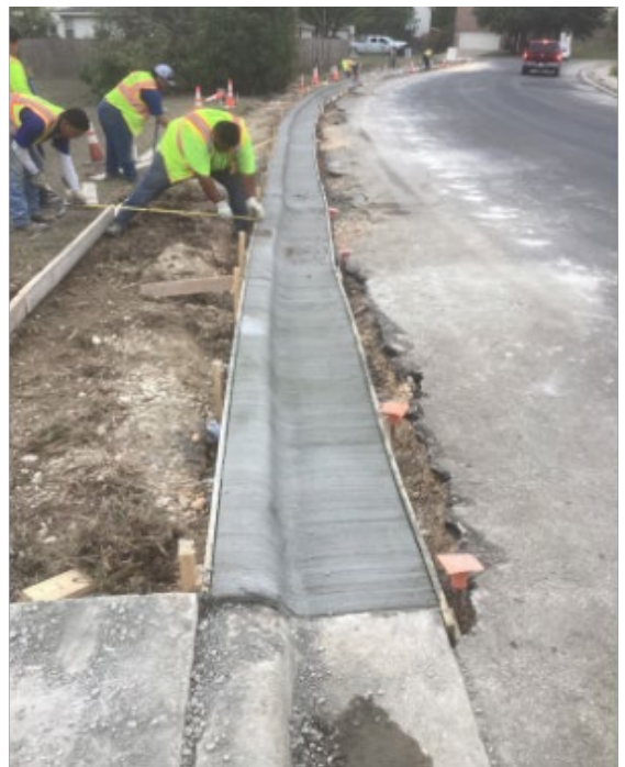
Curb and Gutter Installed / Measuring for Sidewalk
