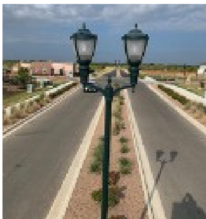
Electrical Work on Masonwood Drive
