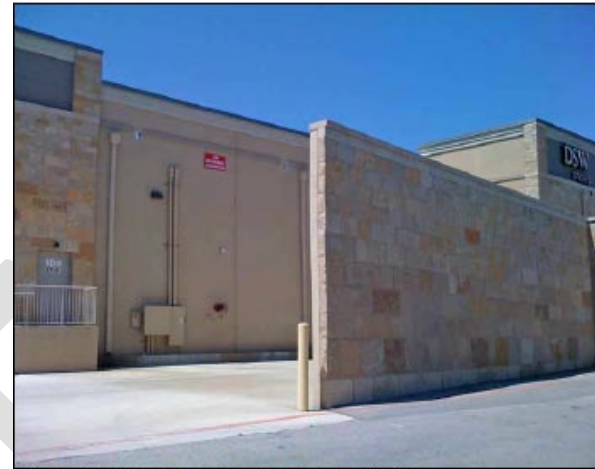
Wing wall used to screen loading dock
