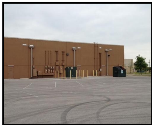
Example of unshielded utility and waste disposal areas
