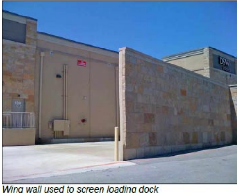
Wing wall used to screen loading dock
