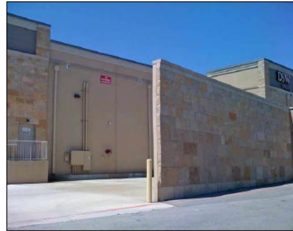
Wing wall used to screen loading dock
