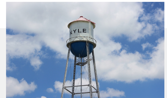
KYLE WATER TOWER
