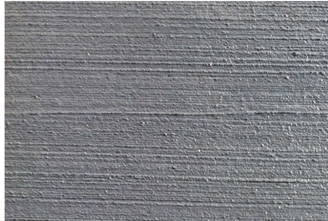
BROOM FINISHED CONCRETE
