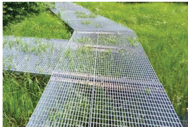
STEEL MESH WALKWAY
