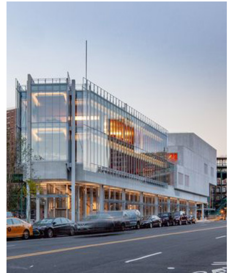
Hotel / Convention Centers can be integrated into retail areas for mutual support. Location: New York City, NY
