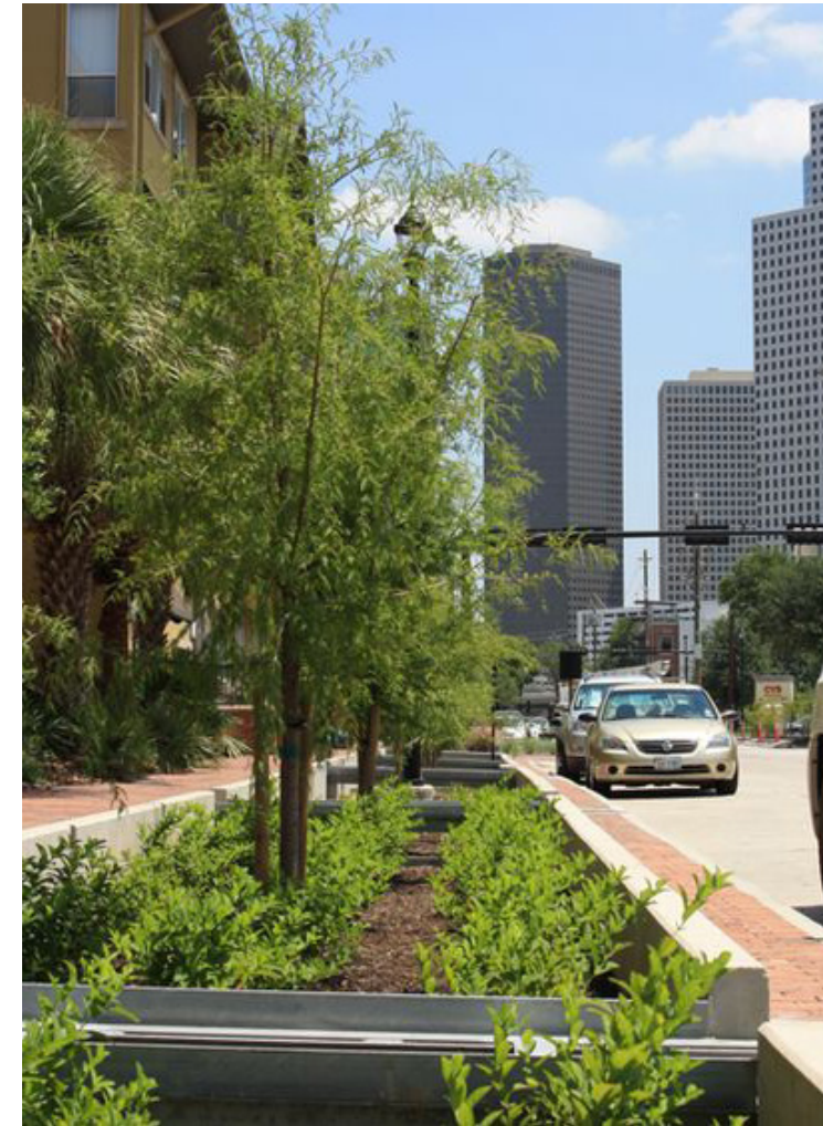
Bioswales and rain gardens help reduce the risk of flooding in the event of a heavy rain and improve water quality
