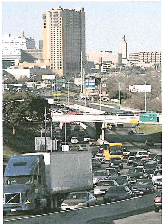
IH 35 looking northbound, 2012
