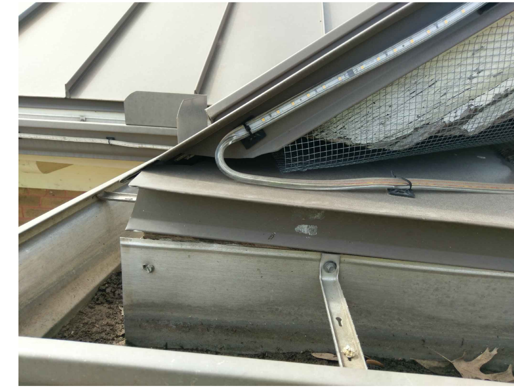
IMAGE 4: WOOD: WOOD FASCIA AT THE RAKE OF THE ROOF APPEARS TO BE THE RESULT OF FAILING PAINT AND AGED, DETERIORATED WOOD FASCIA. DETERIORATED AND WEAKENED WOOD ABOVE THE SOFFITS PROVIDES AN ACCESSIBLE ENTRY POINT FOR RODENTS, INSECTS AND BIRDS. ALSO, DETERIORATED WOOD FASCIA HAS RESULTED IN LOCALIZED SEPARATION OF THE GUTTER ASSEMBLY.
