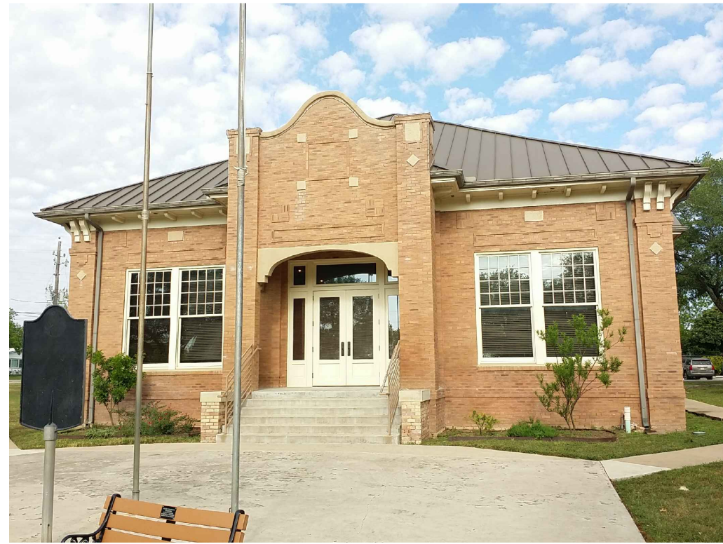
IMAGE 1: EAST ELEVATION: 1. EFFLORESCENCE WAS DETECTED AT THE BASE OF WALL THAT LIKELY OCCURRED DUE TO PROXIMITY OF SPRINKLERS. 2. PILASTER BRICK AND MASONRY CAP DISPLAYED SIGNIFICANT DAMAGE WITH OPEN AND FAILING MORTAR JOINTS. 3. WOOD SOFFITS ARE SAGGING AND IN SOME INSTANCES PULLING AWAY FROM ADJOINING STRUCTURE.
