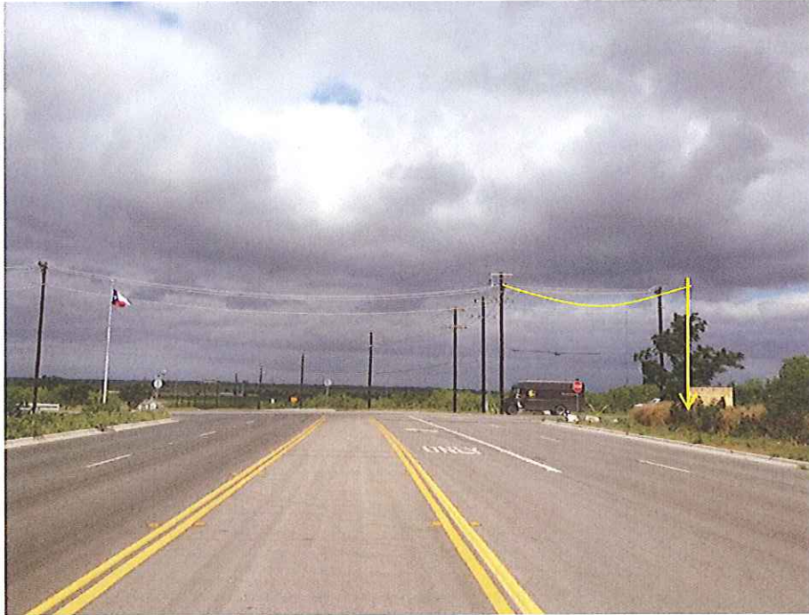
Kyle Crossing/Kohler's Crossing Intersection – Facing West
