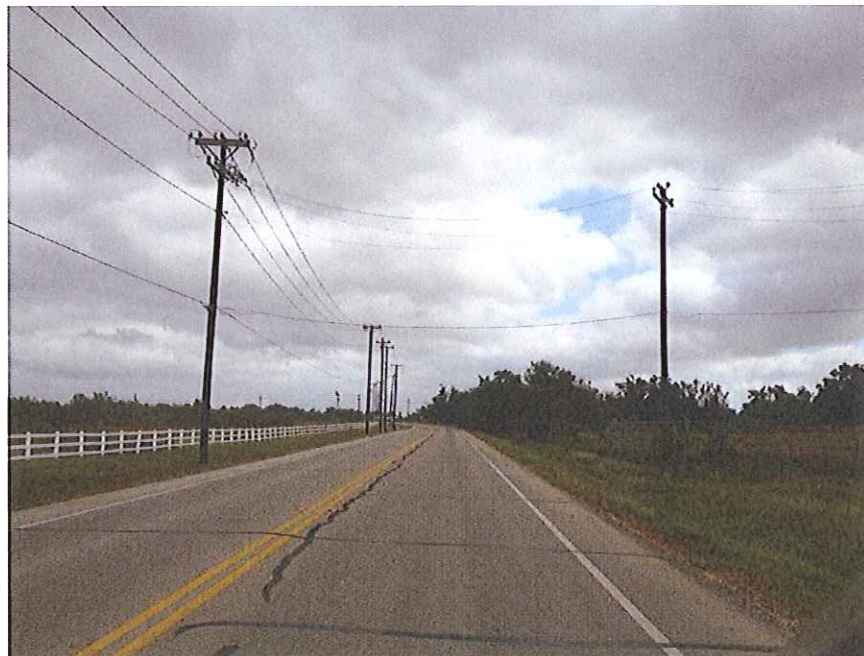
Kyle Crossing overhead electric east-west crossing south of site
