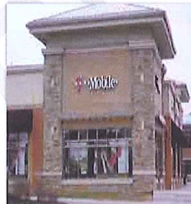
This single-story commercial building has similar detailing on all visible walls.
