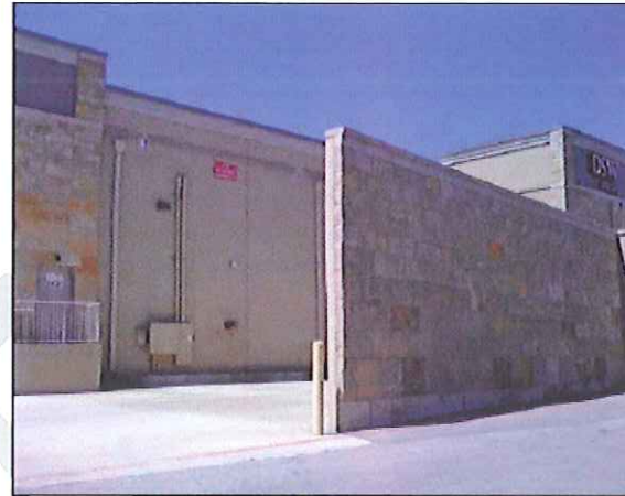
Wing wall used to screen loading dock
