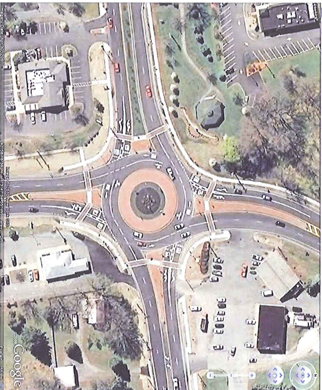
Dunning Street (SR 9) – Malta, New York (Image from Google Earth)
