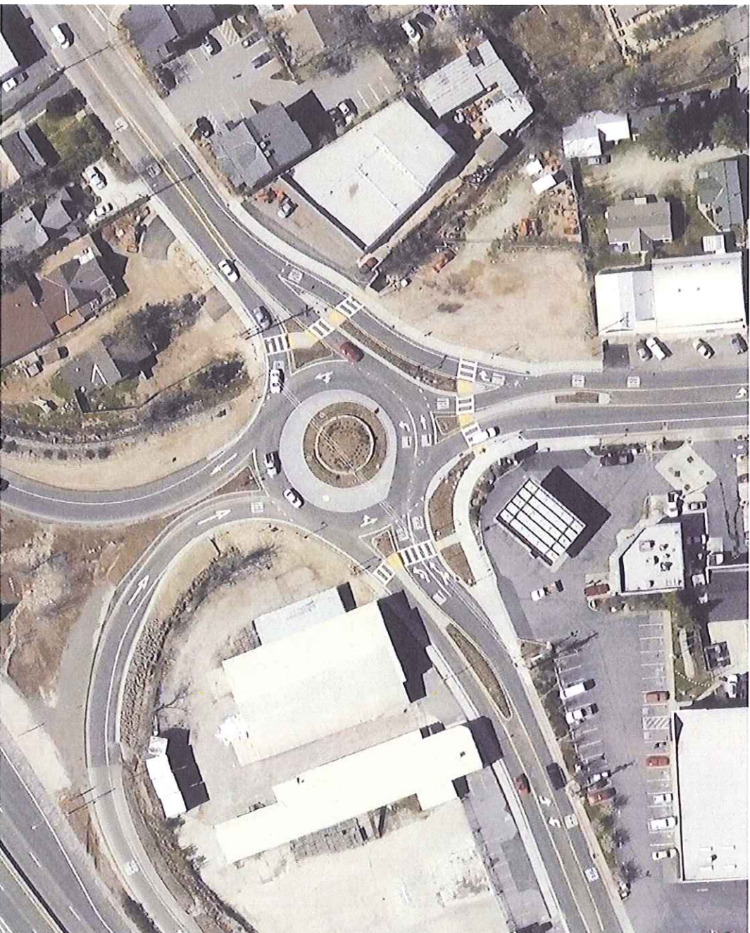
East Main/Idaho/Maryland Road/SH 20 Ramps Roundabout – Grass Valley, California (Image courtesy of Reid Middleton)
