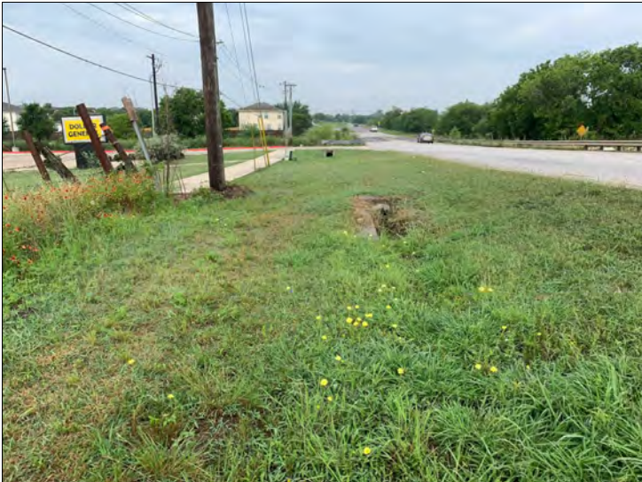
17. Looking west along the south roadside ditch.
