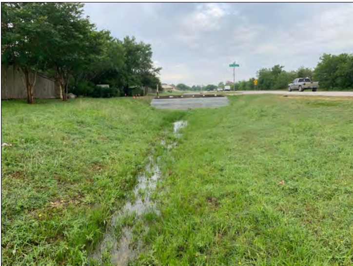
11. Looking west along the roadside ditch towards Indian Paint Brush Dr.
