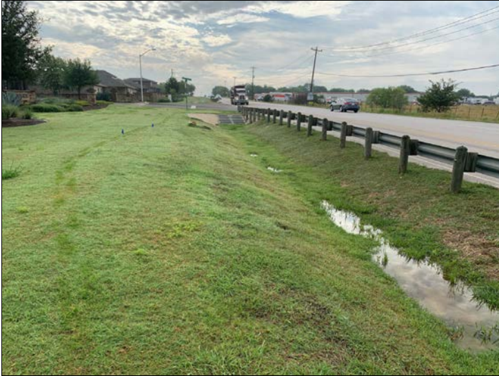
21. Looking east along roadside ditch towards Purple Martin Ave.
