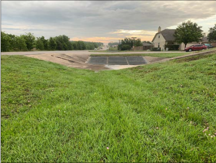
3. Looking west at culvert under Cherrywood St.
