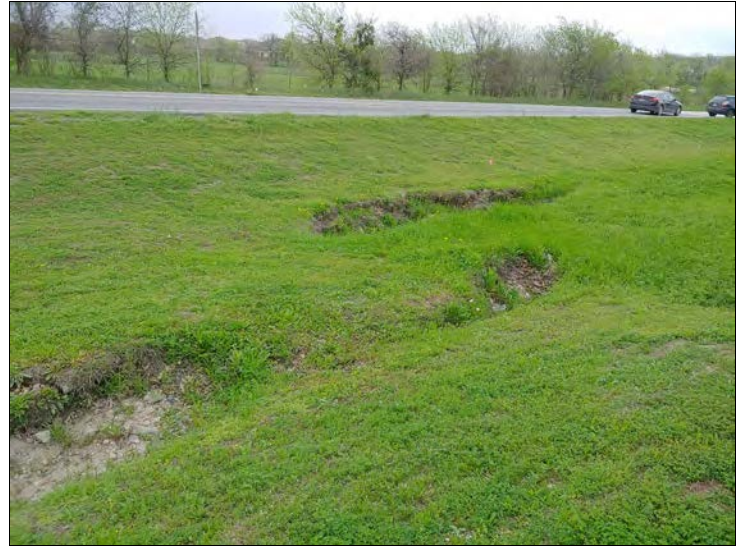
8. For comparison: Another photograph taken by FLT in March 2020. Erosional features typically remain dry except after significant runoff events.
