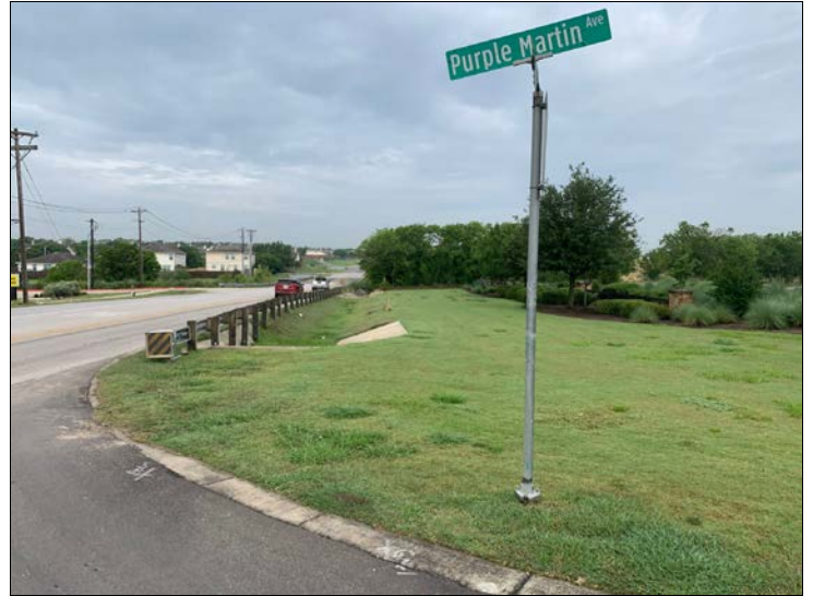
20. Looking west along the roadside ditch from near Purple Martin Ave.
