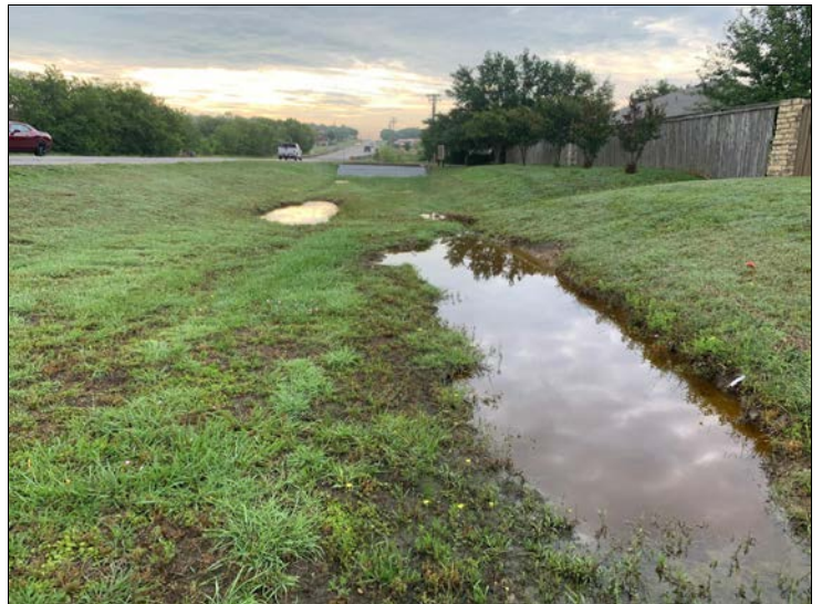
6. Looking east along roadside ditch. Erosional features pond water after significant runoff events.
