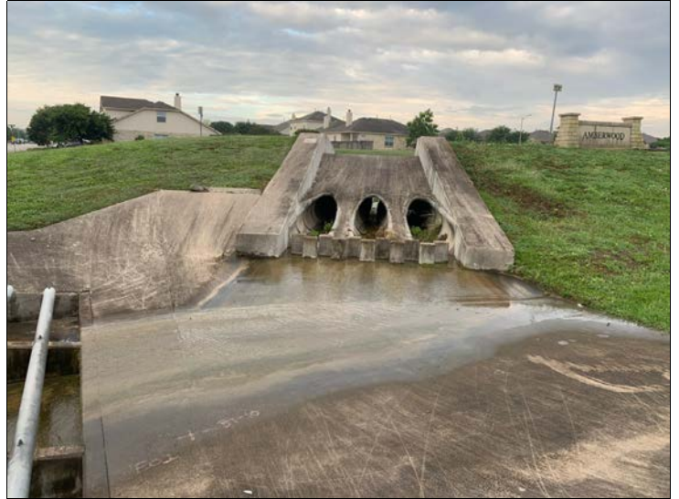
4. Looking south at Amberwood detention pond outfall at the roadside ditch.
