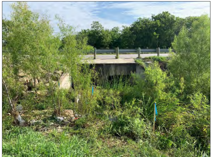
30. Looking north at Richmond Branch bridge.
