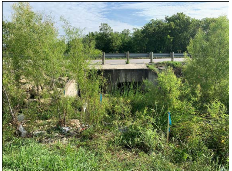
30. Looking north at Richmond Branch bridge.
