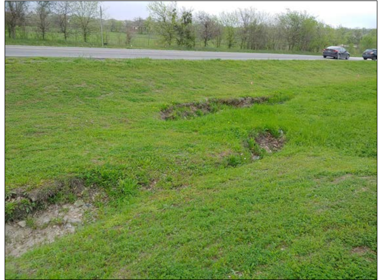
8. For comparison: Another photograph taken by FLT in March 2020. Erosional features typically remain dry except after significant runoff events.
