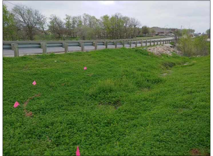
14. For comparison: Photograph taken by FLT in March 2020 showing typical, dry conditions of the roadside ditch between Indian Paint Brush Rd. and Richmond Branch.
