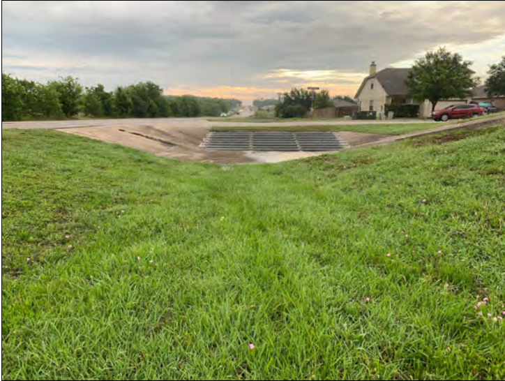
3. Looking west at culvert under Cherrywood St.
