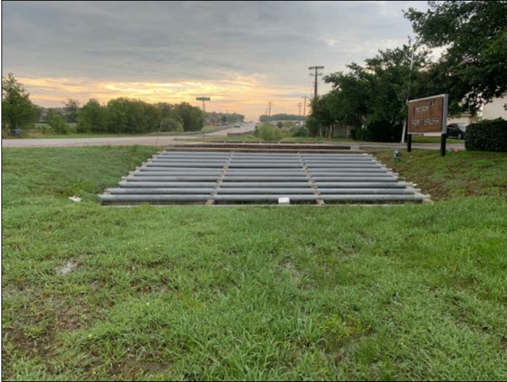
9. Looking east at culvert under Indian Paint Brush Dr.
