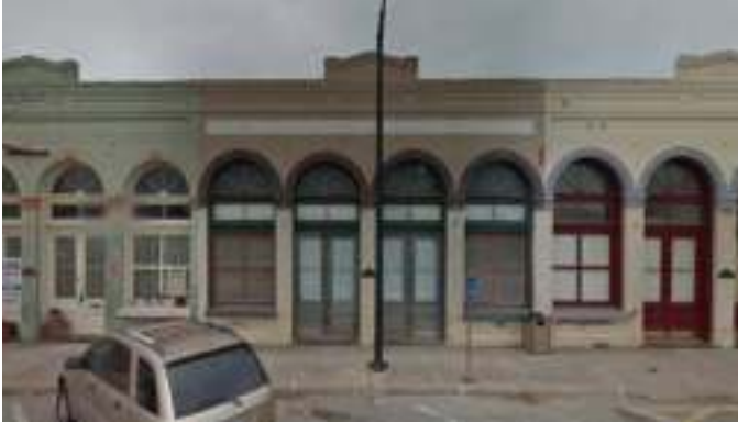
Before: Small Building on East Street, Built in 1893
