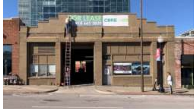
Before: Space being used as Small Parking Garage, built in 1920's
