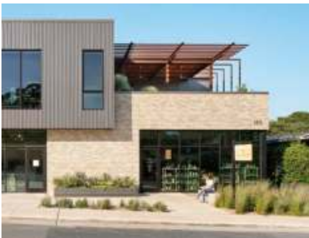
1211 E. 11th Street, Furman + Keil Architects
