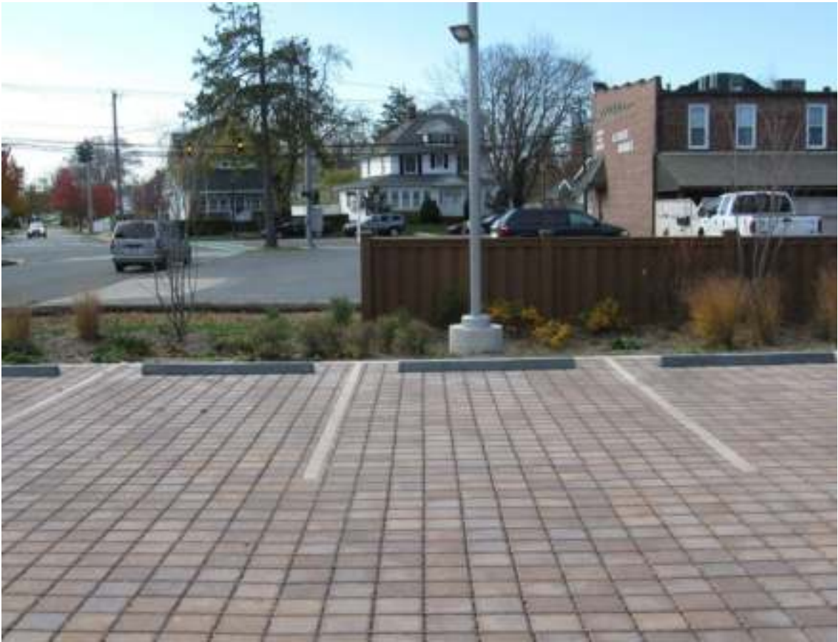
Parking area utilizing permeable paving system
