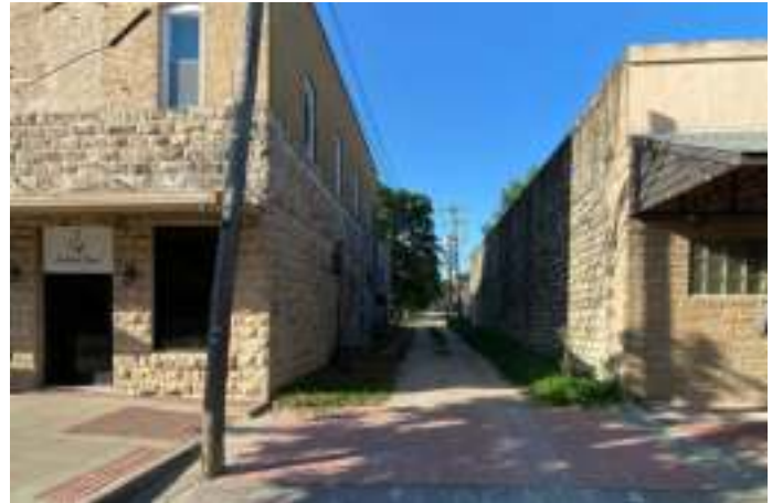
Center Street Alleyway Condition - Before
