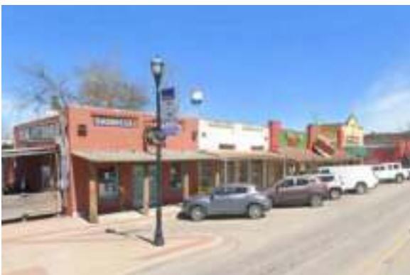
Buildings along north Center Street
