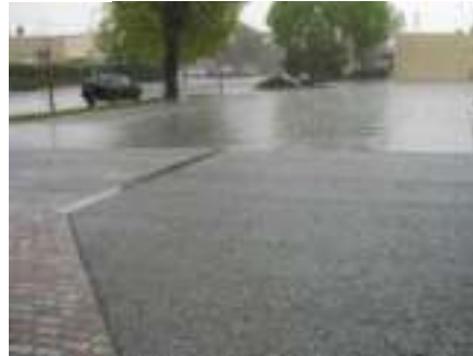
Pervious Asphalt and Concrete Pavers
