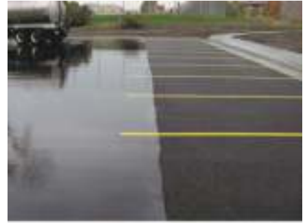
Normal Asphalt (left), Pervious Asphalt (Right)
