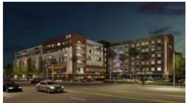
First Point Apartments, Architects Orange
