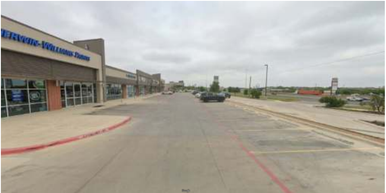
Typical Existing Condition Along Frontage Road
