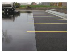
Normal Asphalt (left), Porous Asphalt (Right)
