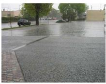
Pervious Asphalt and Concrete Pavers
