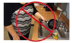
The second most common cause of problems in the treatment system or collection system are related to fats, oils or greases, commonly called FOG. These substances coagulate into large gooey masses, which can negatively impact water treatment plant operations. They can also clog the sewage line leading out of your home.
